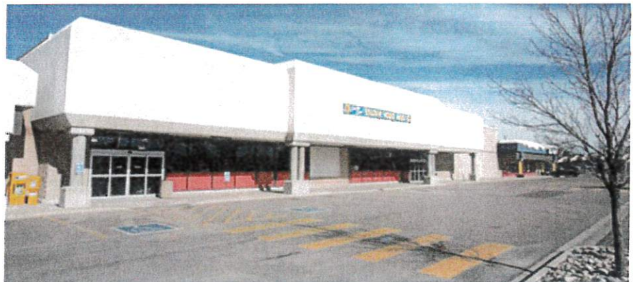
BEFORE: Adaptive Reuse Program - "Renovate Now"
